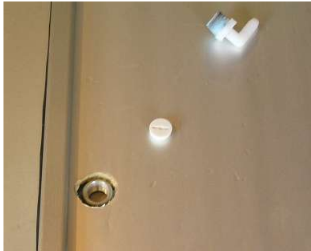
Figure 12: Protective cover removed from SunDrum collector inlet
