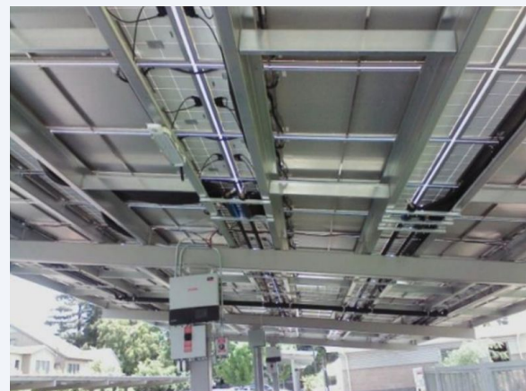
Collectors Visible Under Carport
