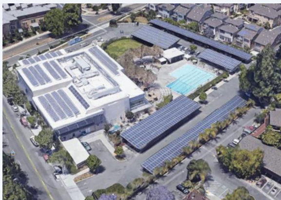
Existing Lodge Carport PV Arrays
