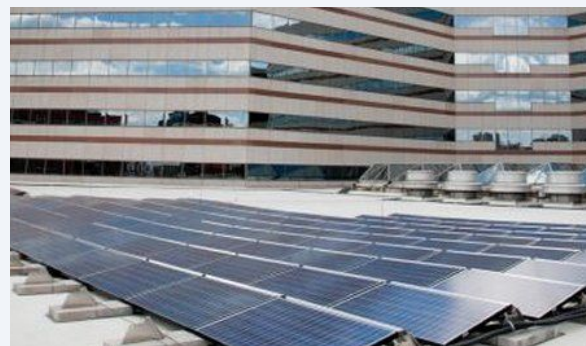
Building Solar Installation
